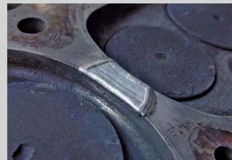
Repairing a water cooled cylinder head of Aluminium (Photo: L&A Lasertechnik, Radebeul)
